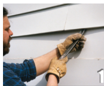
Siding carefully removed
