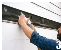
Insulation installed
