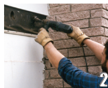
Small holes are drilled
